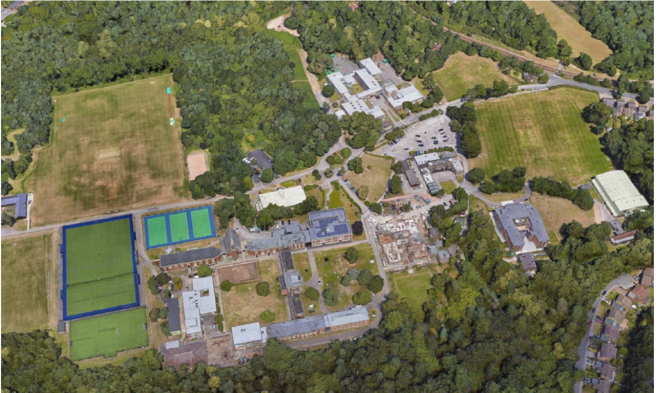
Figure 3: Aerial view of the Royal Russell School campus
