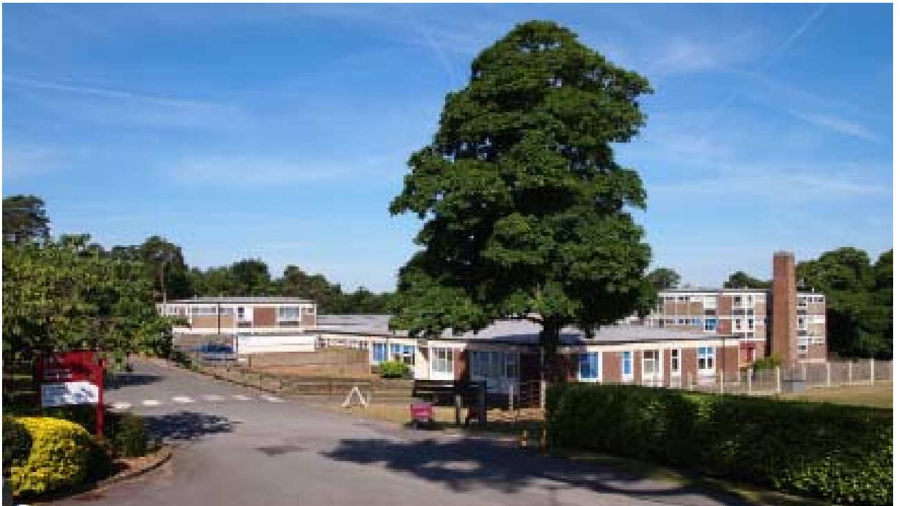
Figure 5: Existing Junior School building when viewed from vehicular access into the site
