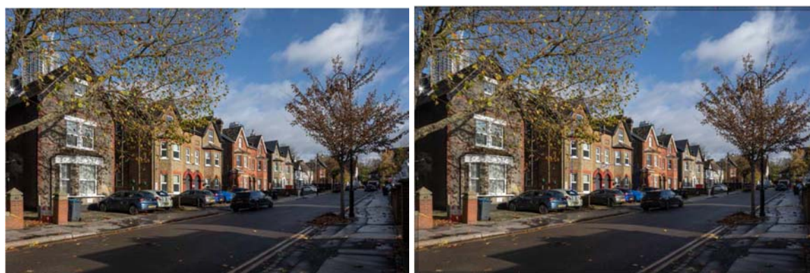
Figures 35 and 36: view from Friends Road looking north-east towards the site without (left) and with (right) proposal
