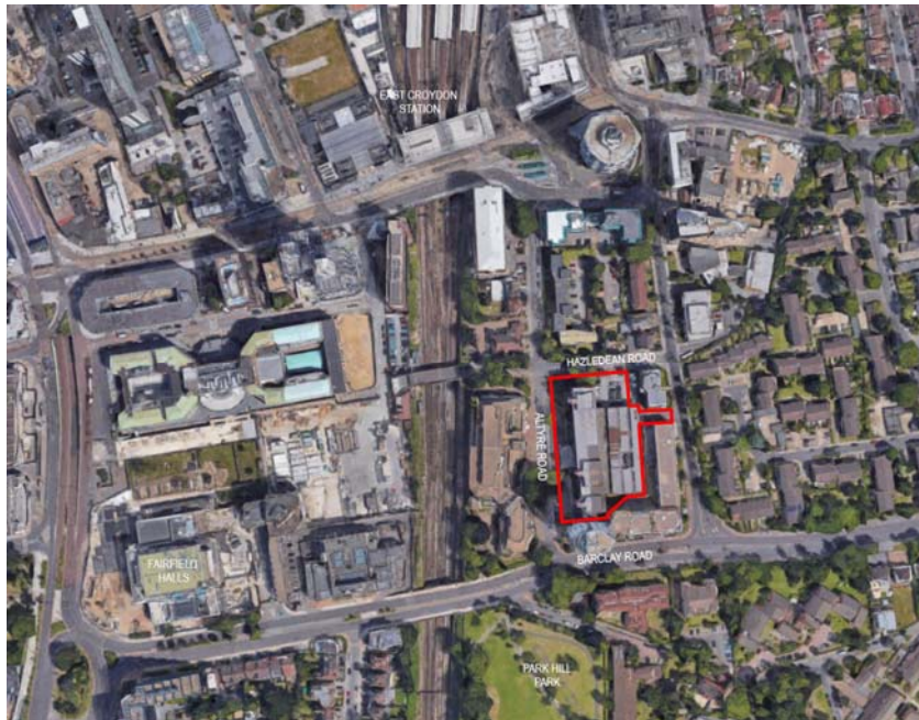
Figure 3: aerial photograph of site in context
