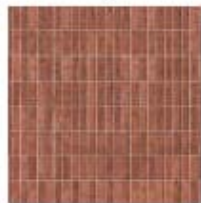
Vertical stack bond brickwork to parapet, above and below windows, and special areas of interest
